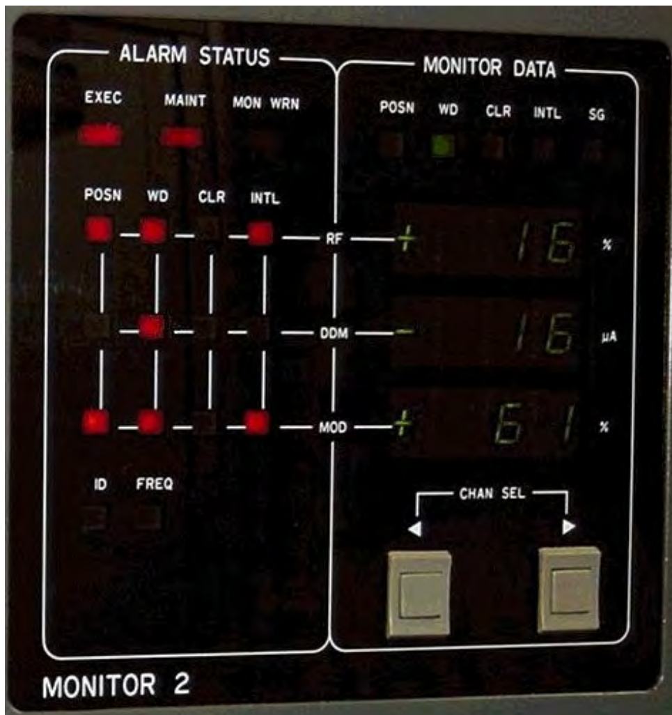
Close up of one monitor panel
